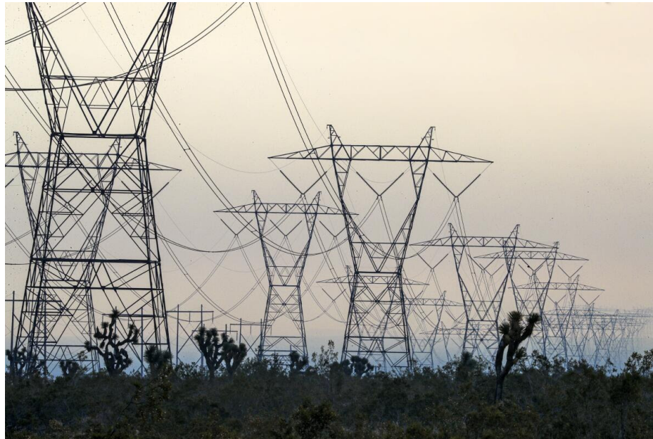
Smoke from the 2020 Bobcat fire casts a pall over power lines running through the Mojave Desert in northern Los Angeles County. (Irfan Khan / Los Angeles Times)
